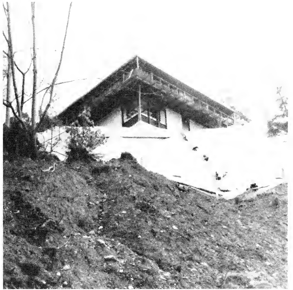
A view of the landslide property showing the house at the edge, the upper part of the slide protected by plastic, and the trees and shrubbery stabilizing the sides of the slide (page 21).
